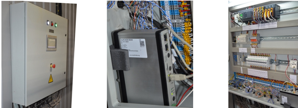
Picture 2 - PLC and myBOX – the hardware basis of the control system.
